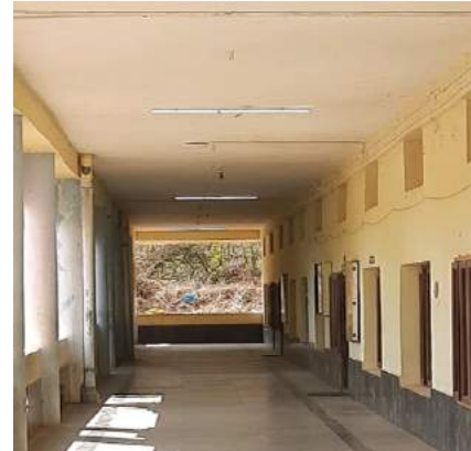
Figure 5 Classrooms opening in to wider corridors with windows and ventilators allowing for better ventilation
