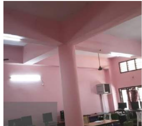
Figure 4 Class rooms with larger windows , open ventilators , led tubelights and painted in light bright colours for better daylight and ventilation
